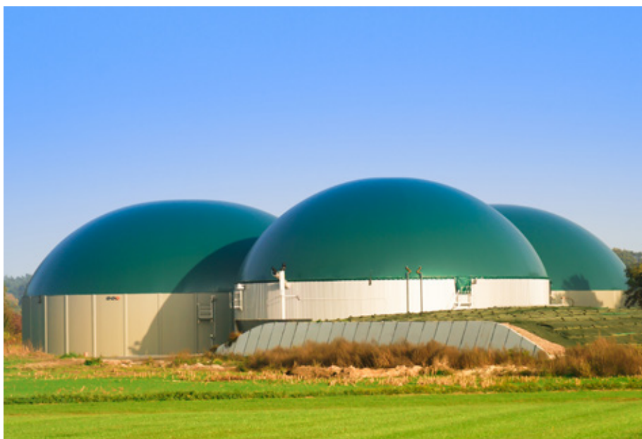
Biogas gas storage in use
